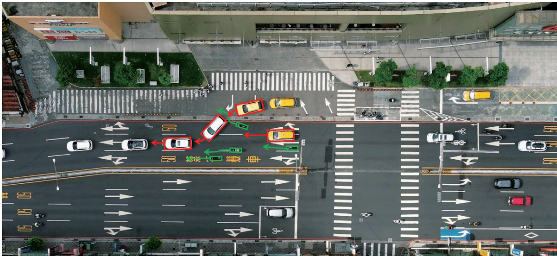
「路外設施進出車流衝突」空拍圖 Aerial view of "Traffic Conflicts Caused by Vehicles Entering or Exiting Roadside Facilities"
