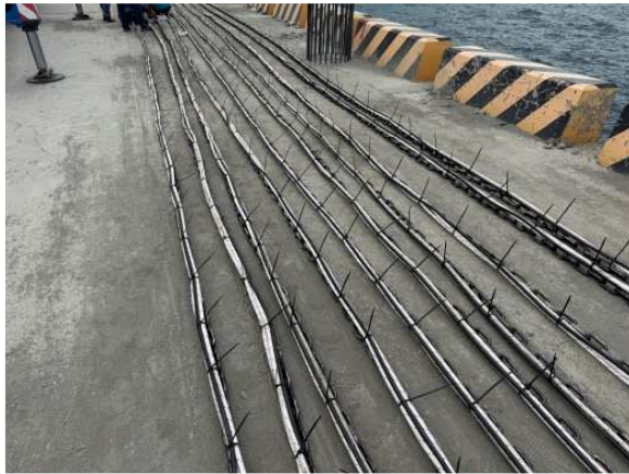
(a) 錨鍊、編織繩及海底電纜綁紮
