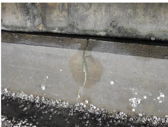
Defect #6 橋墩帽梁混凝土裂縫
