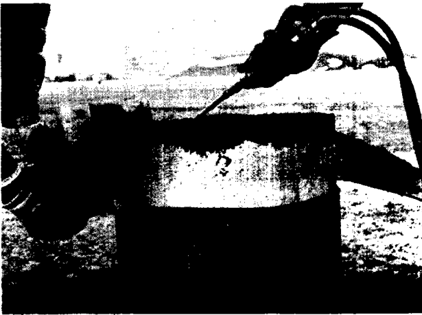
(6) If the coating is hard to pull off, the inside of the pipe is heated to 100 \sim 130^{\circ}\text{C} . It can then be putted off easily.
