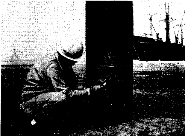
(3) The edges of the coating are removed.
