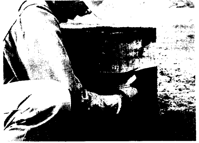
(7) The edge of the coating is removed.
