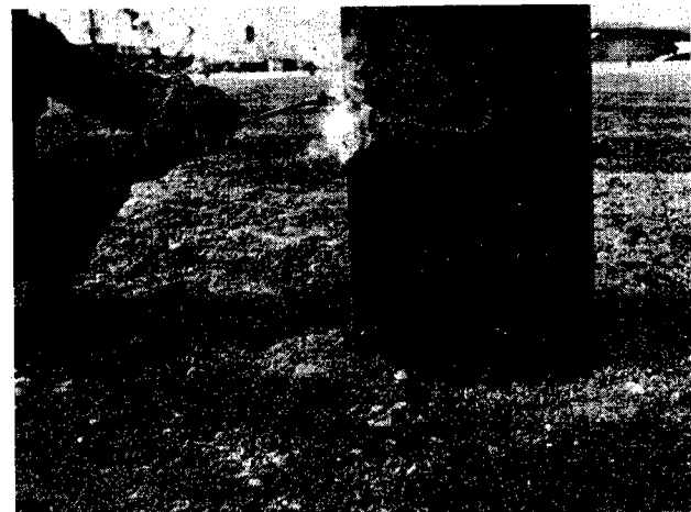
(3) Cutting is done by an acetylene burner.
