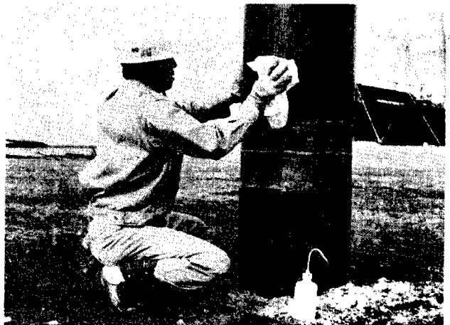
(4) Dirt and grease on the coating are removed with an organic solvent.
