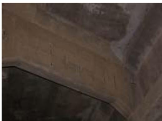
T15-05 間隔梁鋼筋腐蝕外露
