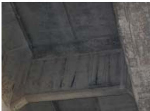
T2-08 間隔梁鋼筋腐蝕外露
