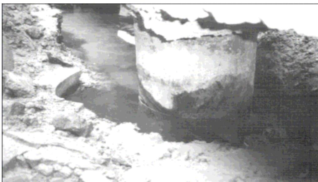
圖 2-1 Kobe 港在土壤液化時未損壞之棧橋基樁(Finn and Fujita 2002)
