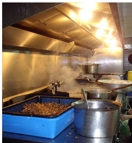
B1廚房瓦斯器具未設置漏氣遮斷閥
