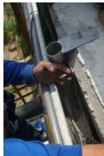
(3) 鎖固側邊面板膨脹螺絲
