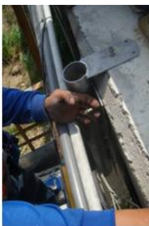
(3) 鎖固側邊面板膨脹螺絲
