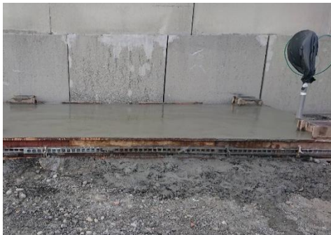
(c)混凝土澆置
