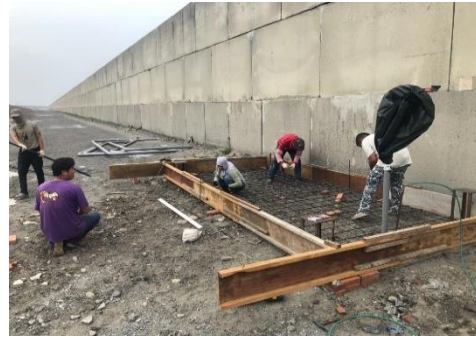
(b)鋼筋綁紮
